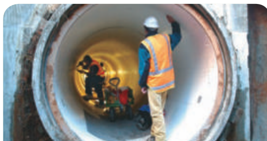
Upgrading existing stormwater treatment devices
