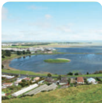
The Mangere Wastewater Treatment Plant will reach its flow capacity in about 2027, at projected population growth rates
