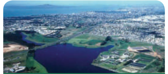
The Rosedale Wastewater Treatment Plant is a state of the art facility which treats flows from North Shore City
