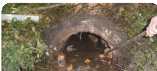
If flows in pipes get too low, like during the 1994 drought, problems with solids settling occurs
