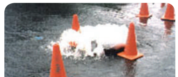
It is not possible to prevent all overflows occurring
