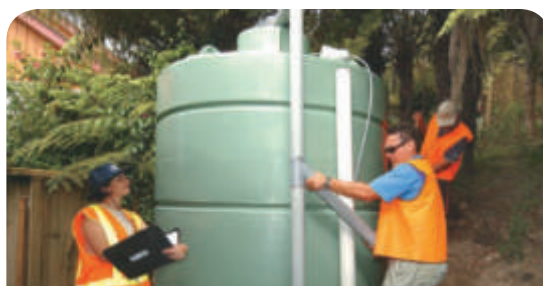
Retrofitting storage tanks
