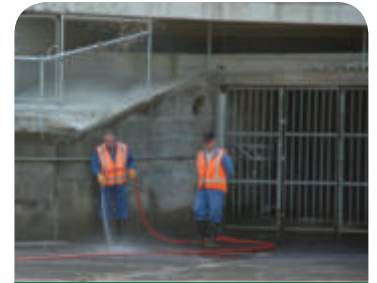
Unpleasant odours from any part of wastewater systems
