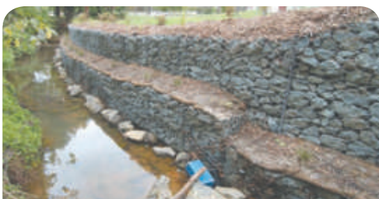
Stream protection works
