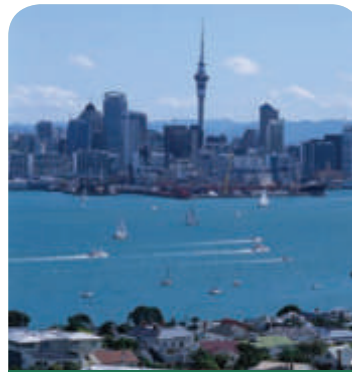
Some major sewers are near or at capacity in Central Auckland and some cannot be maintained because they flow full for significant periods of time
